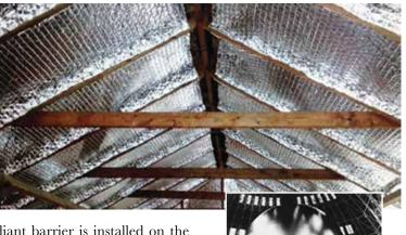
diant barrier is installed on the rafters in the attic, much of the heat radiated from the hot roof is reflected back toward the roof allowing for a cooler attic.
