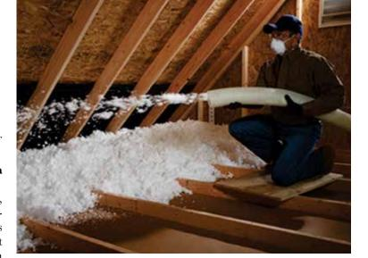
the type of insulation to be used and where it will be used. Make sure that each type of insulation is listed by R-value. Beware of any contract or verbal offering that quotes the job in terms of thickness only (e.g. "14 inches of insulation"). Remember, it is the R-value, not the thickness that tells how well a material insulates. Avoid contracts with vague language such as R-values with the terms "plus or minus;" "+ or -;" "average;" or "nominal."
