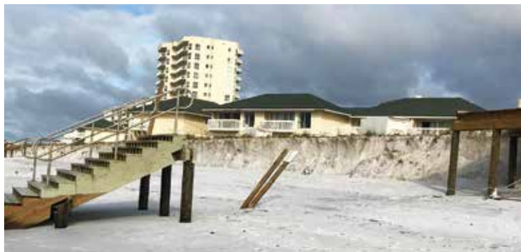
Hurricane Sally. The action was later ratified by the Destin City
