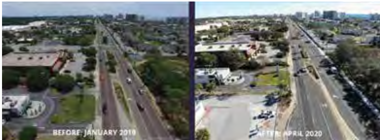
Before and after: these photos, near Gulf Shore Drive, show the new bicycle lanes and damaged sidewalks replaced.
